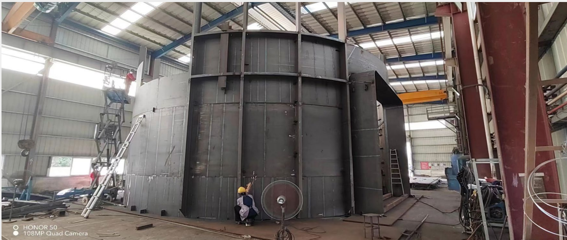
Steel plate work, Asia
