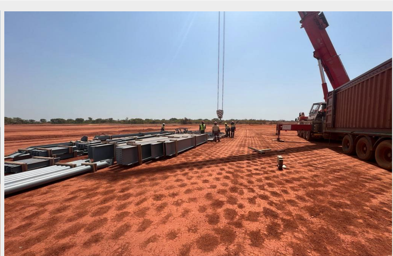
Unloading of the first steel on site
