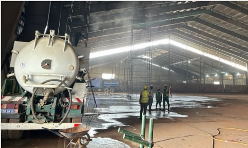
Shed cleaning in readiness for DSO
