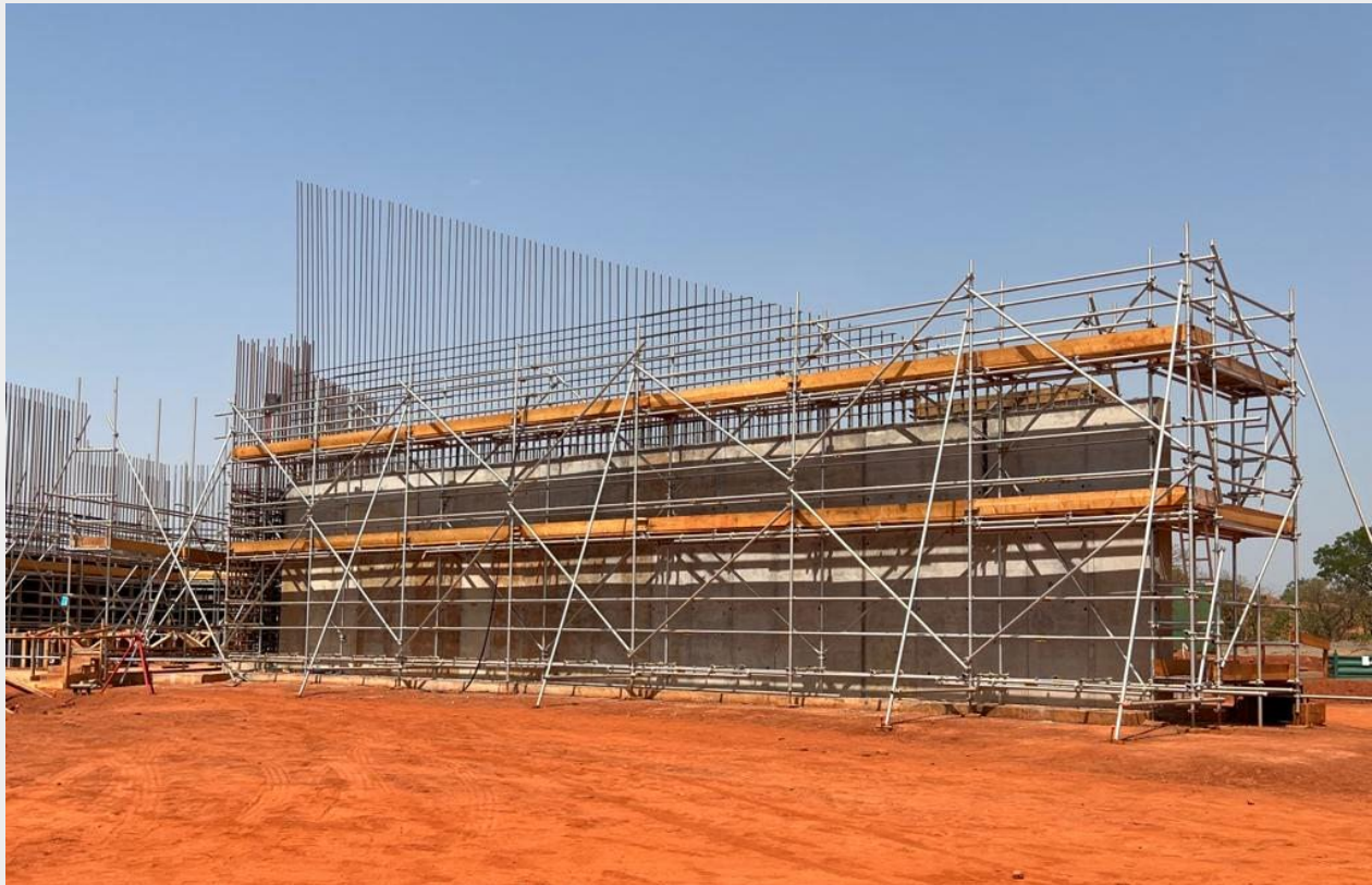
Primary crusher wall scaffolding
